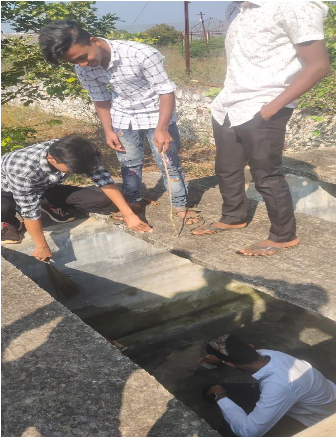
Water sump being cleaned during campus cleaning.
